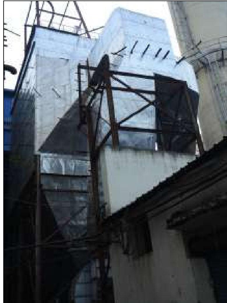
ESP for 75 TPH Boiler Capacity
