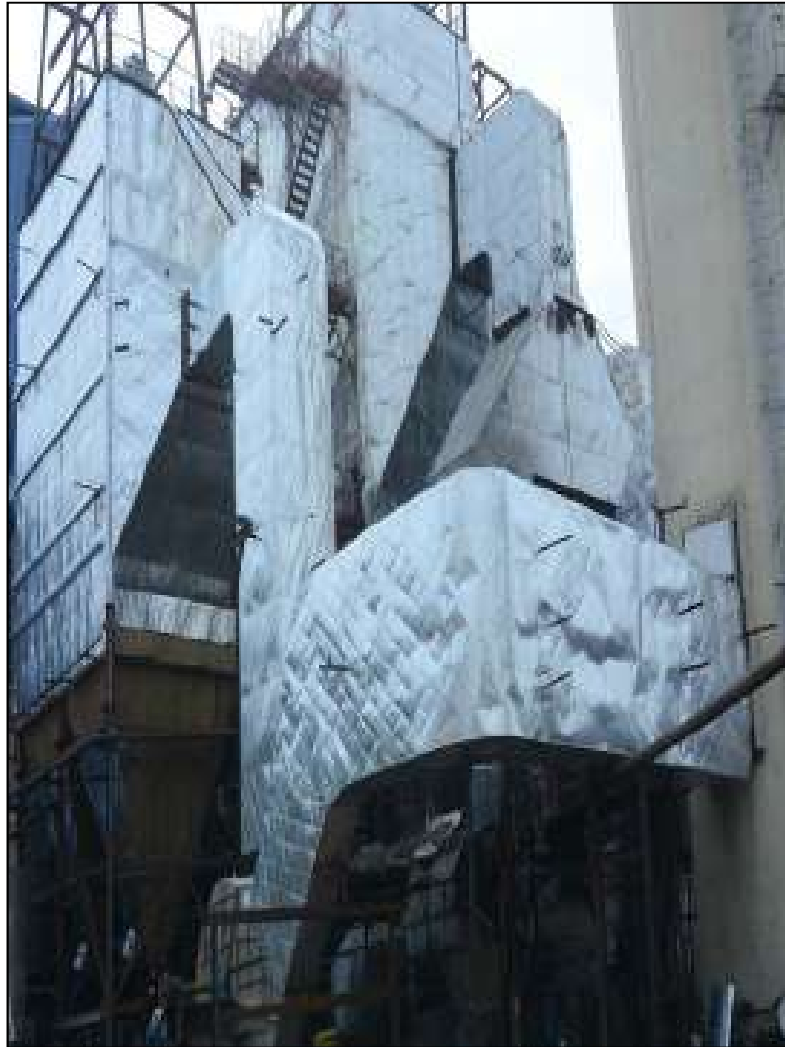
ESP for 20 & 90 TPH Boiler Capacity
